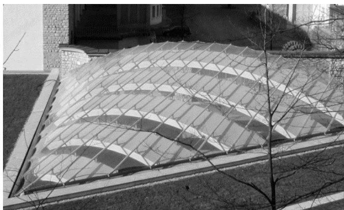
Fig. 3: E-ON Info Center Walchensee Power Plant in Kochel, 2001, ETFE-film single layer structure, mechanically pre-stressed, on aluminum girders and wooden (laminated) arches, NOWOFOLON ET6235 200 \mu\text{m} , 1 field, total surface area: approx. 391 \text{m}^2 , architect: HAUSCHILD & BOESEL, Munich, Structural Design and Engineering: DITTRICH, München, ENGINEERING+DESIGN, Linke & Moritz GbR, Rosenheim, realization membrane roof: COVERTEX GmbH, Obing [3]
