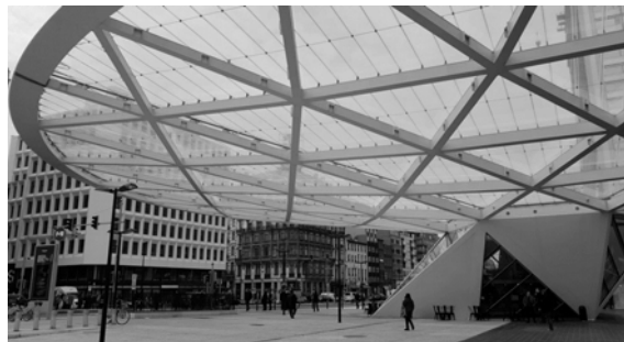
Fig. 5: Place Rogier, Brussels, 2018, ETFE-film, single layer structure, mechanically pre-stressed, NOWOFOLON ET6235 250 µm, 3 fields, total surface area: approx. 3000 m 2 , architect: Xaveer De Geyter Architects (XDGA), Brussels, membrane engineering: KONSTRUCT AG, Rosenheim, realization membrane roof: TAIYO EUROPE GmbH, Sauerlach, Foto [5]
