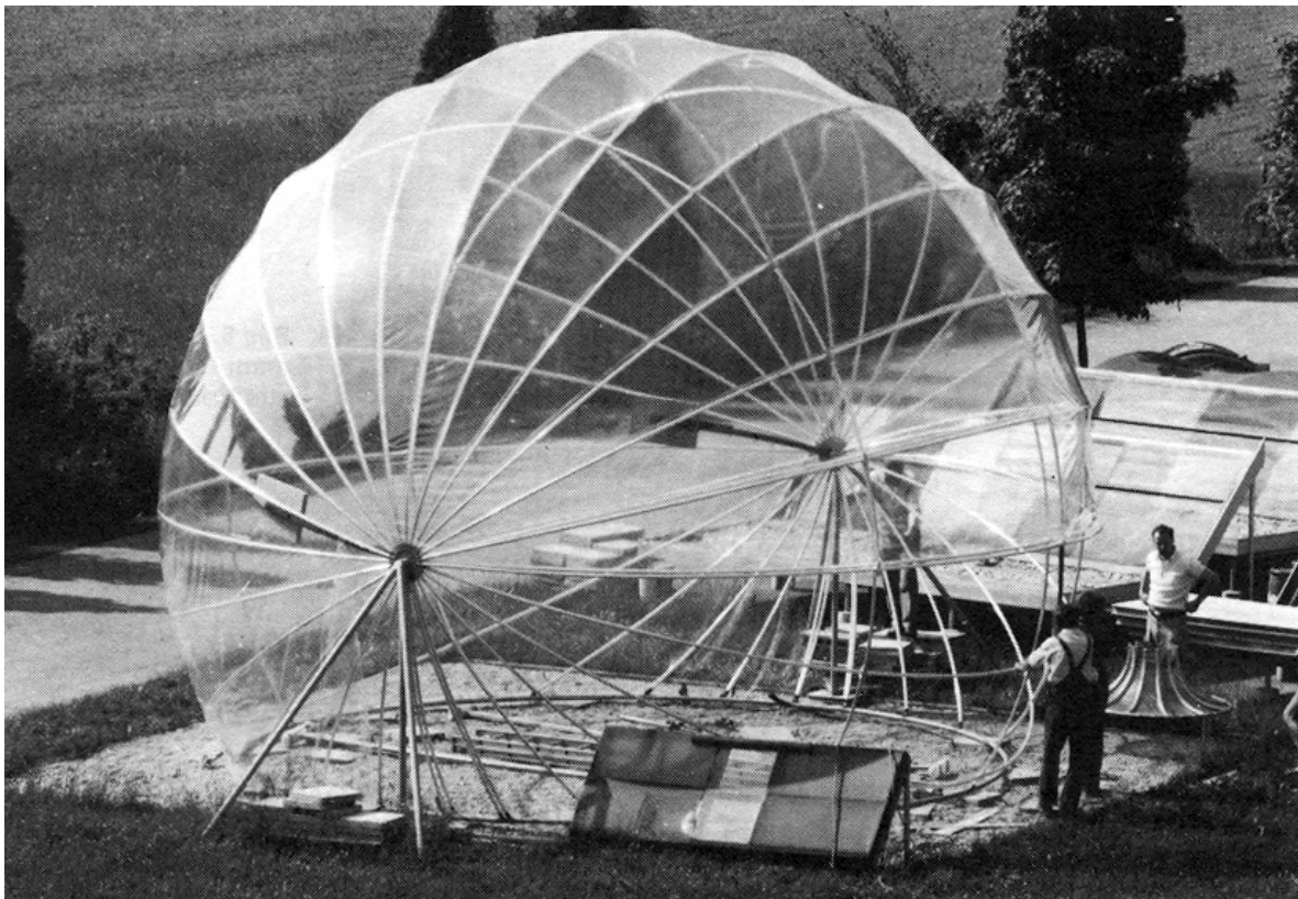
Fig. 1: ETFE-Sphere, temporary, 3 rd Internationale Sun-Forum, Hamburg, 1980, ETFE-film, single layer structure, mechanically pre-stressed in combination with slim bended rods, HOECHST HOSTAFILON ET 150 µm, max. distance of the rods approx. 1,0 m, sphere diameter approx. 8 m, height approx. 6 m, Design: Hans and Jürgen KLEINWÄCHTER, BOMIN SOLAR RESEARCH, Lörrach, Execution: Herbert KOCH, KOIT GmbH, Rimsting [4]
