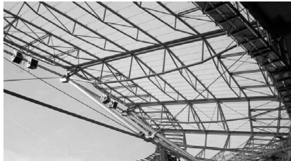
Fig. 4: AWD Arena (today: HDI Arena), Hanover, grandstand roof, 2005, ETFE-film single layer structure, mechanically 4pre-stressed, cable- and girder-supported, NOWOFOLON ET6235 250 µm, 34 fields, total surface area: approx. 10.000 m 2 , architect: SCHULITZ + PARTNER GmbH, Brunswick, Structural Design and Engineering: RFR Ingenieure GmbH, Stuttgart, WEYER Beratende Ingenieure im Bauwesen GmbH, Dortmund, ENGINEERING+DESIGN, Linke & Moritz GbR, Rosenheim, realization membrane roof: WEYSS & FREYTAG Ingenieurbau AG [3], [6]
